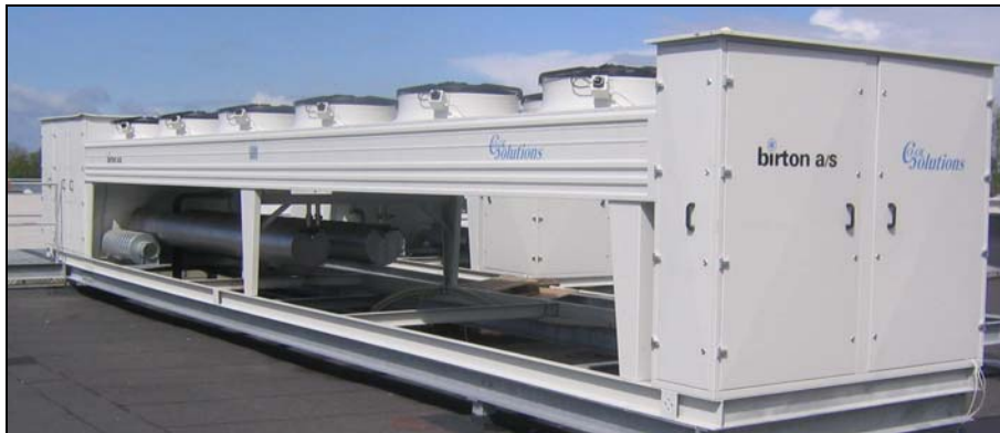
A picture from the installation
