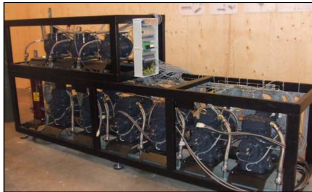
A picture from the installation
